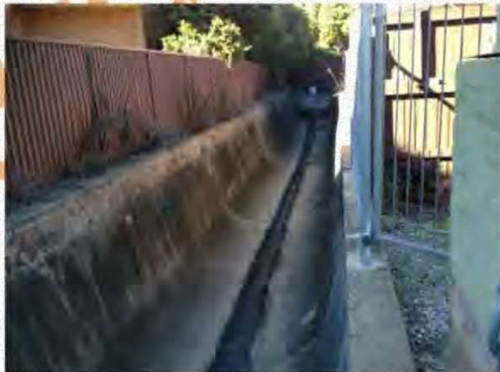
Photo 1: Powells Creek water level gauge at Elva Street
