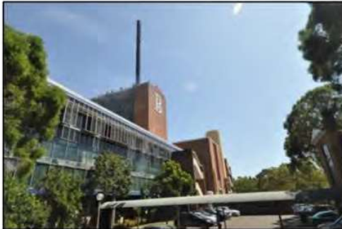
Figure 31. View of the covered walkway joining the eastern façade of the factory to the administration building.
