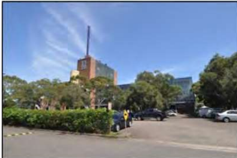
Figure 29. View west encompassing a detail of the factory's eastern façade and open-air car park.
