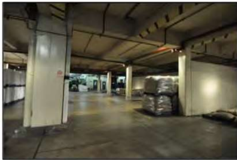
Figure 39. Detail of space located on the lower ground floor. (Source: Heritage 21, 09.03.16)
