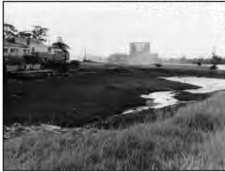
Figure 11. Bushells Factory, c. 1966, without chimney. 21
