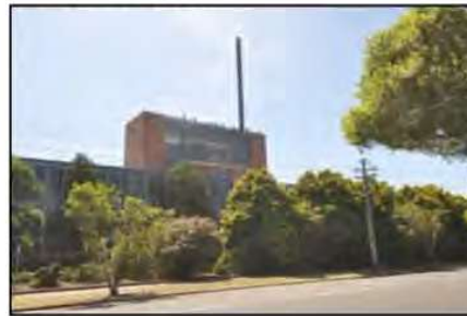
Figure 26. View towards the subject site from Burwood Road. (Heritage 21, 09.03.16)
