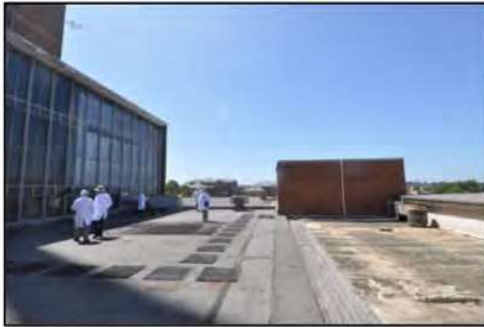
Figure 37. Roof space located on second floor.
