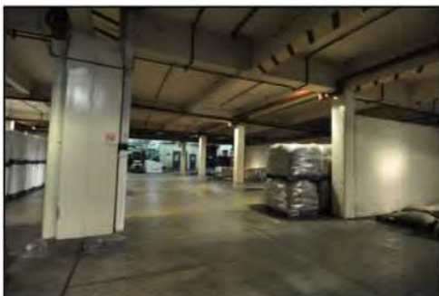
Figure 35. Detail of space located on the lower ground floor.
