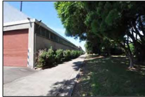
Figure 32. Western façade of the factory with landscaped area located along the western boundary evident on the right.
