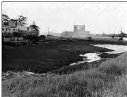
Figure 15. Bushells Factory, c. 1966, without chimney. 33
