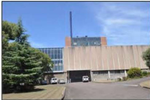
Figure 35. Detail of northern façade of factory with precast concrete panels. (Source: Heritage 21, 09.03.16)
