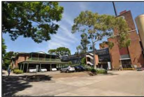
Figure 31. View south-west encompassing the northern façade of the administration building and a detail of the eastern façade of the factory. (Source: Heritage 21, 09.03.16)
