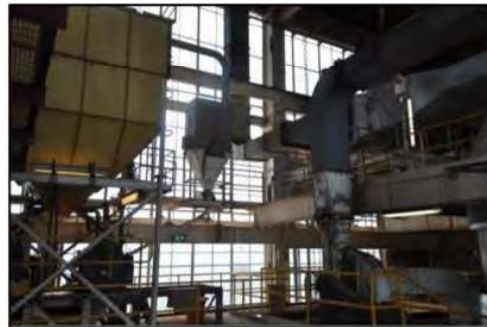
Figure 48. View looking up of the roasting hall from fifth floor platform.
