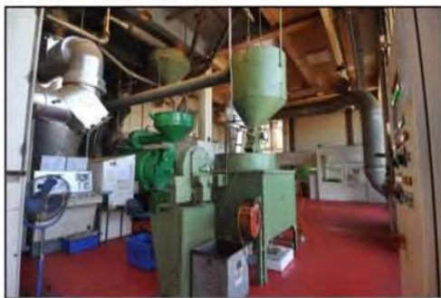
Figure 41. Detail of space and equipment located on second floor. (Source: Heritage 21, 09.03.16)
