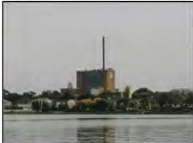
Figure 23. View of subject site from Hen and Chicken Bay, c. 2007. 65
