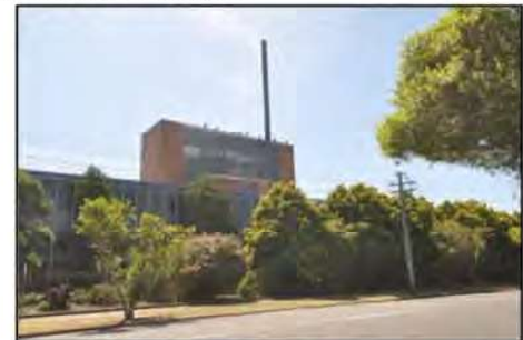
Figure 30. View towards the subject site from Burwood Road. (Heritage 21, 09.03.16)
