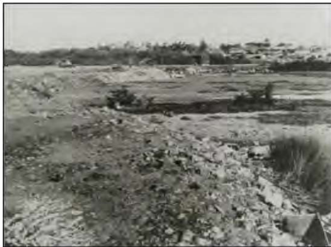
Figure 11. Reclamation works at Exile Bay, c.1930. 27
