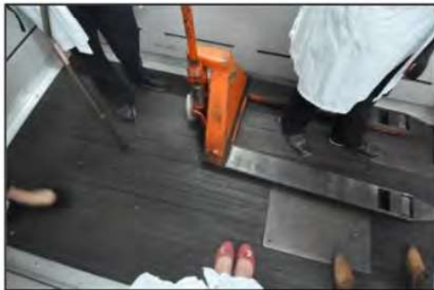
Figure 49. View of timber floored service lift. (Source: Heritage 21, 09.03.16)
