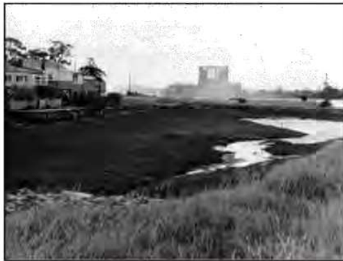
Figure 11. Bushells Factory, c. 1966, without chimney. 36
