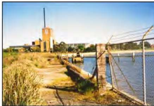
Figure 16. View looking west towards the subject site, c 1991 51
