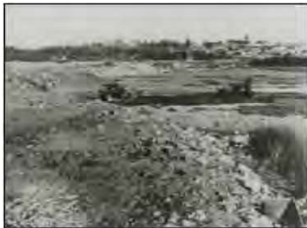
Figure 9. Reclamation works at Exile Bay, c.1930. 15
