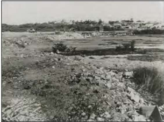
Figure 9. Reclamation works at Exile Bay, c.1930. 30
