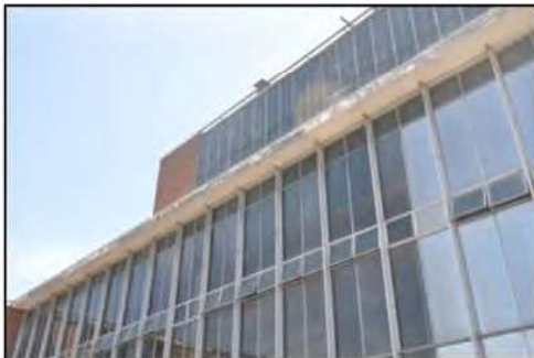
Figure 41. View of clerestory aluminium glazing as viewed from the second-floor roof space.
