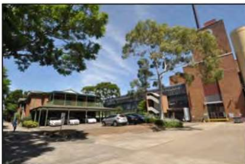
Figure 35. View south-west encompassing the northern façade of the administration building and a detail of the eastern façade of the factory.
