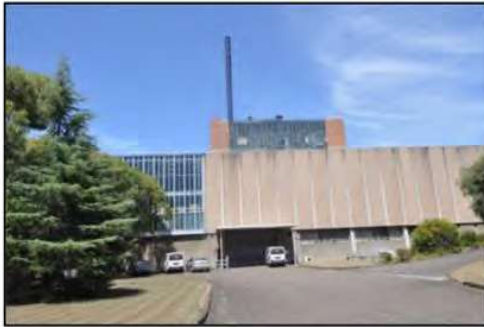
Figure 31. Detail of northern façade of factory with precast concrete panels.
