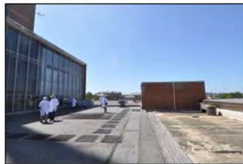
Figure 42. Roof space located on second floor. (Source: Heritage 21, 09.03.16)
