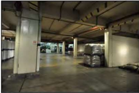
Figure 43. Detail of space located on the lower ground floor.
