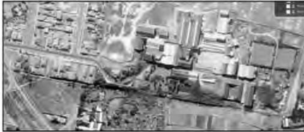
Figure 53. Aerial view of the Davis Gelatine Factory site in 1943. 80
