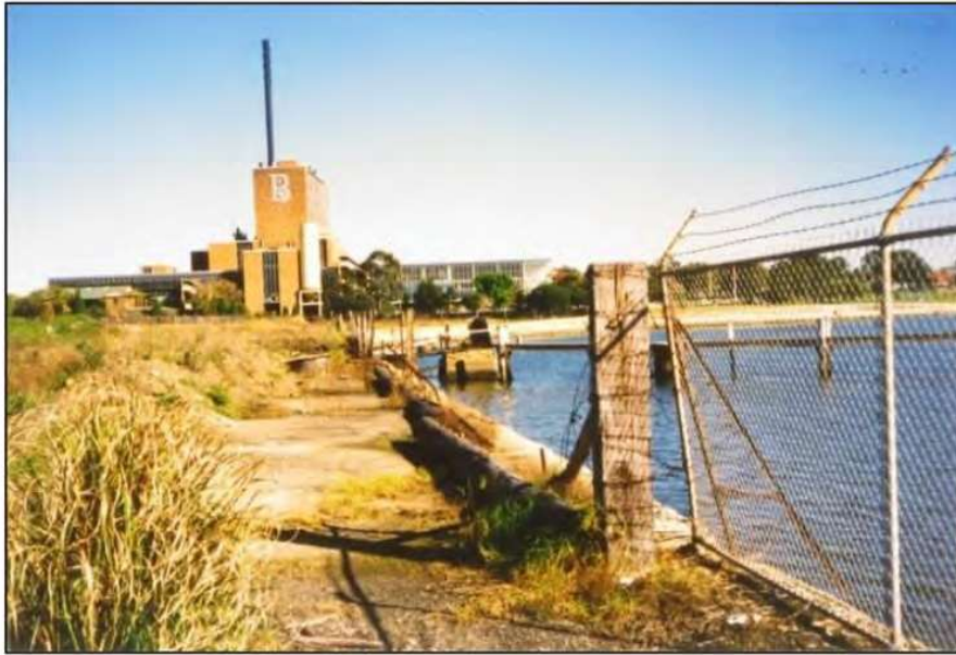
Figure 16. View looking west towards the subject site, c 1991. 36
