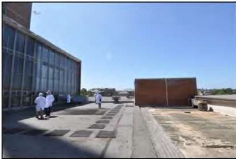
Figure 45. Roof space located on second floor.
