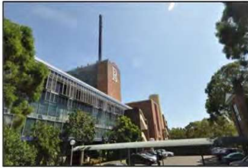
Figure 27. View of the covered walkway joining the eastern façade of the factory to the administration building. (Source: Heritage 21, 09.03.16)
