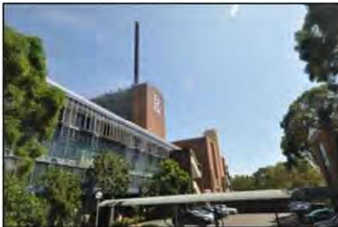
Figure 23. View of the covered walkway joining the eastern façade of the factory to the administration building.
