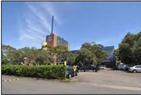
Figure 37. View west encompassing a detail of the factory's eastern façade and open-air car park.
