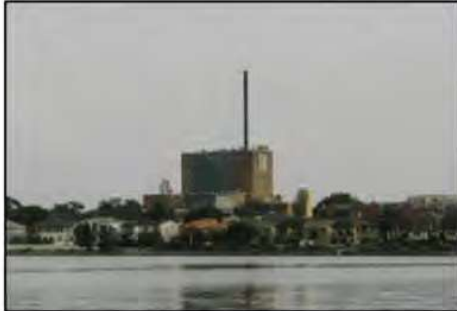
Figure 27. View of subject site from Hen and Chicken Bay, c. 2007. 62
