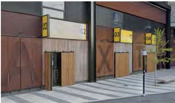
Figure K19-16 Detailed, activated urban services frontage, Caxton Works, London (source: Google Streetview)
