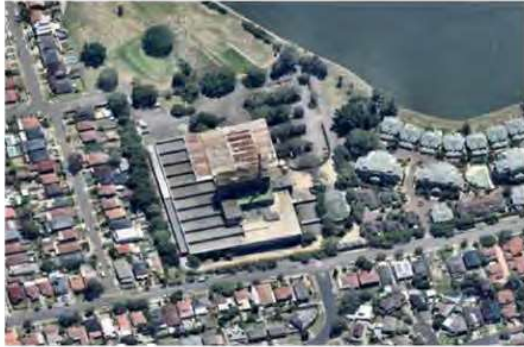
Figure K19-1 Aerial photo (source: nearmap.com)
