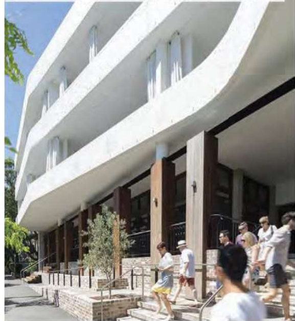
CASBA MIXED USE HOUSING, WATERLOO NEW SOUTH WALES
