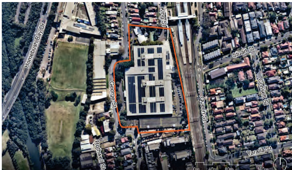
Figure 1.2 The extent of the subject site (outlined in orange) in its local context. (Source: Google Maps 2022 with GML overlay)
