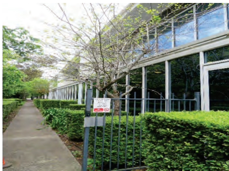
Figure 2.3 The east elevation of the warehouse building.
