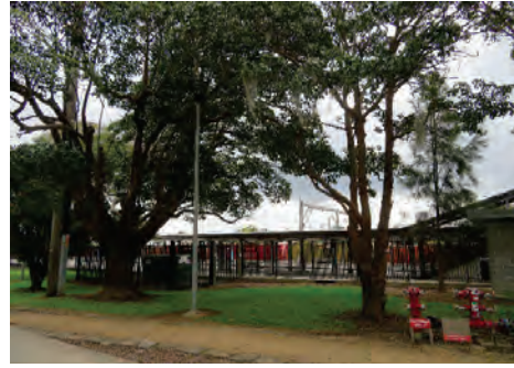
Figure 2.16 View from Concord West Memorial Park across the railway tracks to the subject site.
