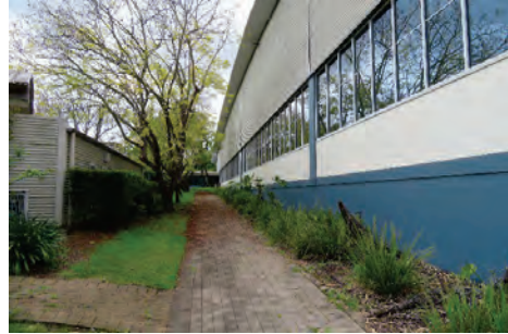
Figure 2.6 View of the north elevation of the building, showing the entrance to the childcare centre to the left.
