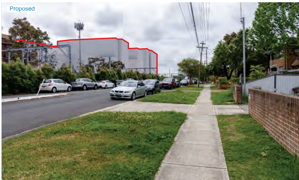
Figure 93 207 Queen St - proposed view from the Visual Impact Assessment, Figure 13 (Ethos Urban, 2023) with a red line added by SGL showing approximate building outline
