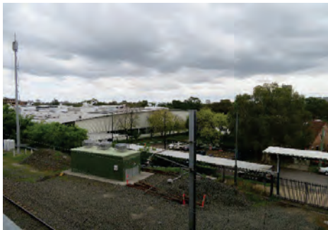
Figure 2.1 View of the site looking southwest from Concord West Station.
