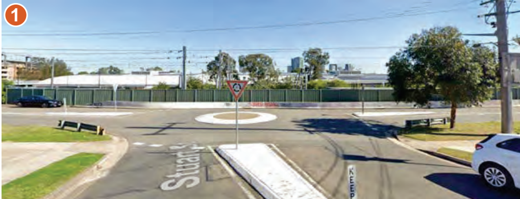
Figure 10 View of the site from Stuart Street, Concord West looking west (Google, 2021)
