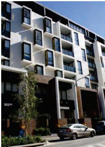
Figure 49 Example of an eight storey apartment building in Harold Park, Forest Lodge with articulated two storey street wall and upper level setback.
