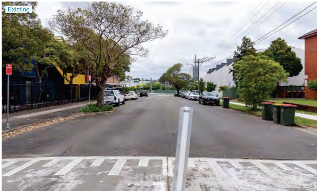
Figure 90 17 Stuart St - existing view from the Visual Impact Assessment, Figure 10 (Ethos Urban, 2023)
