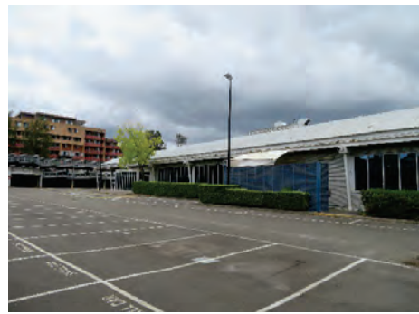
Figure 2.4 View of the east elevation of the building, showing an on-grade carpark in the foreground and the two storey carpark at the rear of the site.
