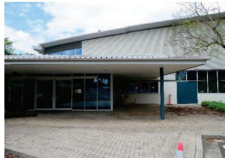
Figure 2.2 The entrance to the call centre on the site.
