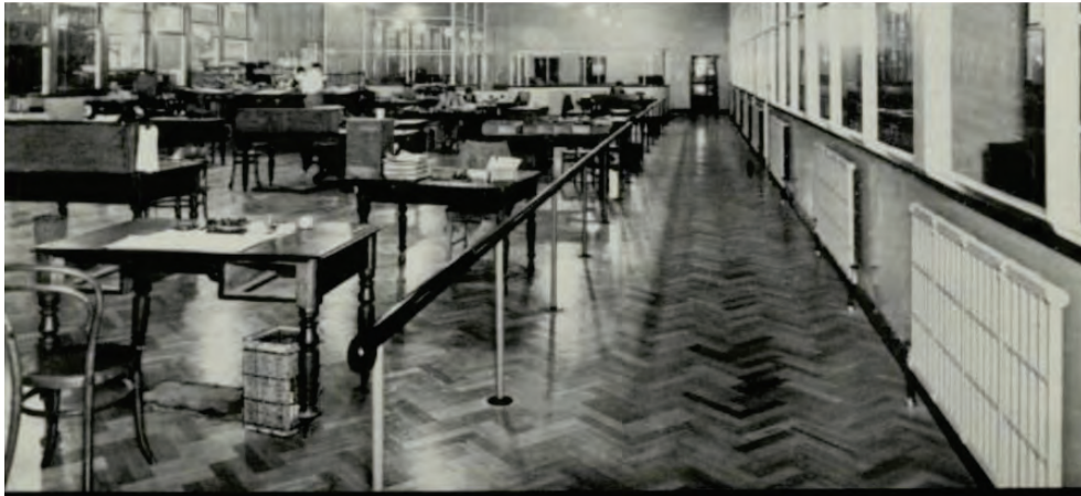
Figure 3.6 The open plan interior of the building with parquetry flooring. (Source: Decoration and Glass , Vol. 3 No. 11 March 1938, p 20)
