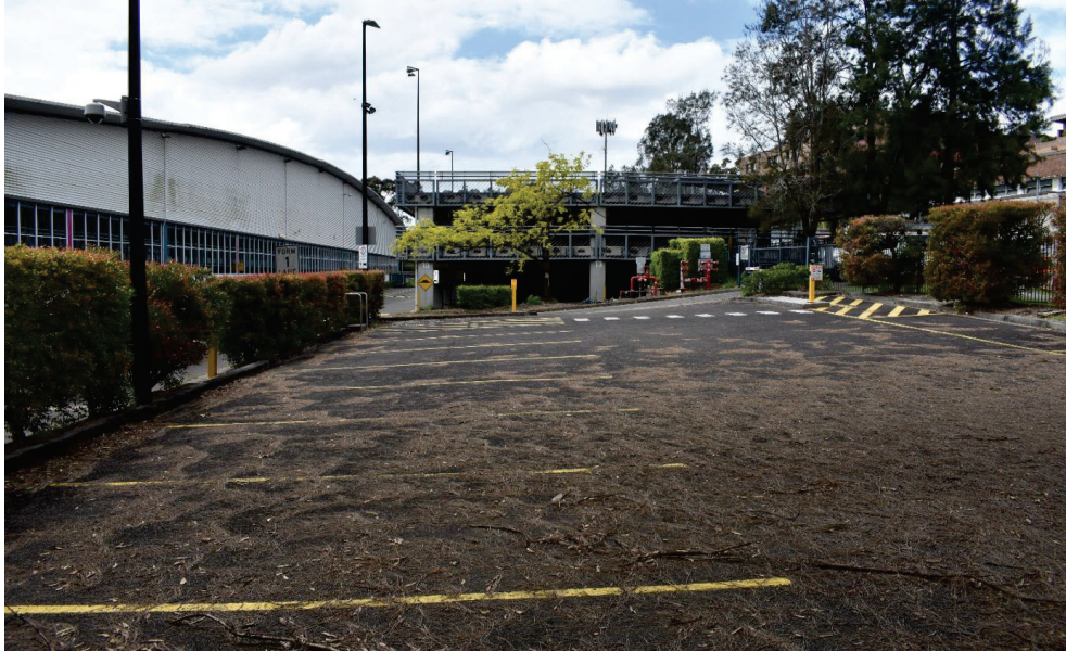
Figure 4.7 Sealed road surfaces and multilevel parking structure in south of study area.
