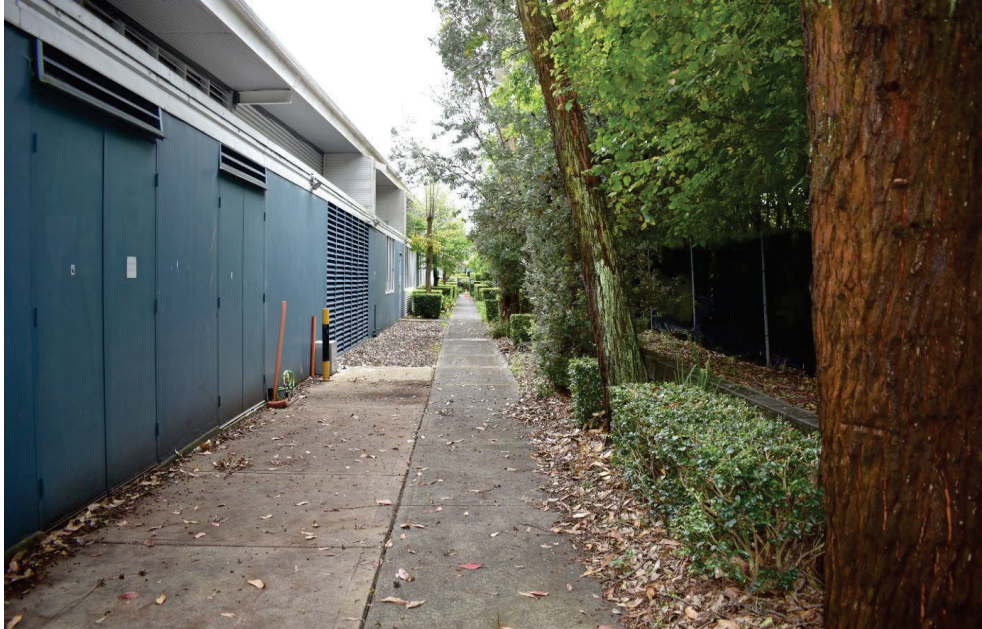
Figure 4.9 Ground surfaces along eastern extent of study area.
