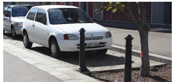
Example of a Living Landscape Blister (with street tree) integrated with street parking
