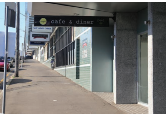
Recent development response to slope on western side of Victoria Road
