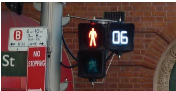
An example of a pedestrian countdown timer in George Street, Sydney (photo source: Sydney Emerald City)
