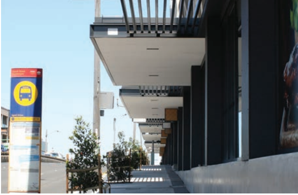
Example of an awning design with 'breaks' and street tree planting at 81-110 Victoria Road
