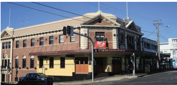
The Lyons/ Victoria Roads intersection creates an opportunity for celebrating the heritage character
