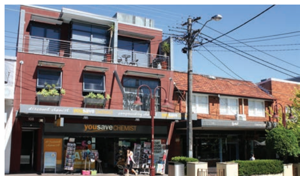
An example of a new 2+1 storey incremental infill
