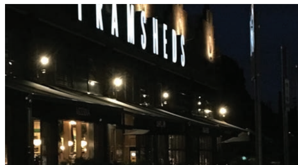
A combination of illuminated signage, uplighting of upper level facade, wall-mounted above awning spot lights and interior lighting on a heritage building
