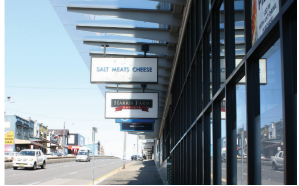
Example of a continuous awning outside Harris Farm, Victoria Road
