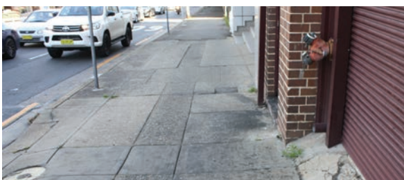
Existing condition of footpath along Victoria Road
