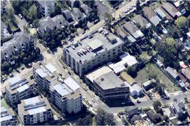
Figure K3-1 Aerial photo (source: nearmap.com)
