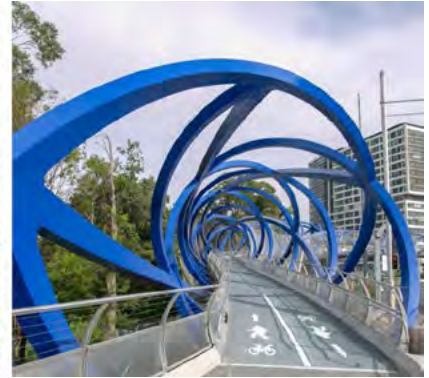
Examples of the bridge design
