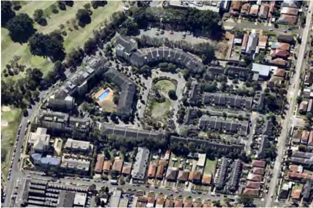
Figure K11-1 Aerial photo (source: nearmap.com)
