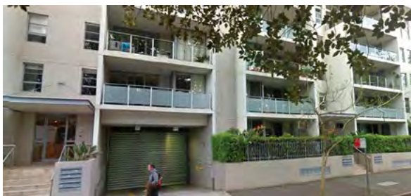
Example of a 'mixed' facade
