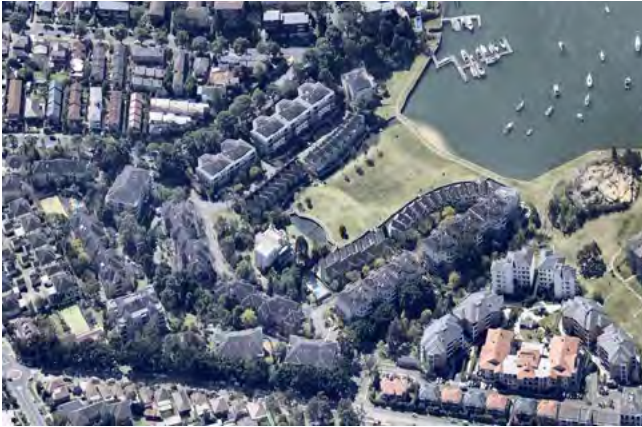
Figure K2-1 Aerial photo (source: nearmap.com)
