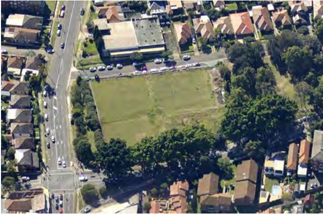
Figure K9-1 Aerial photo (source: nearmap.com)
