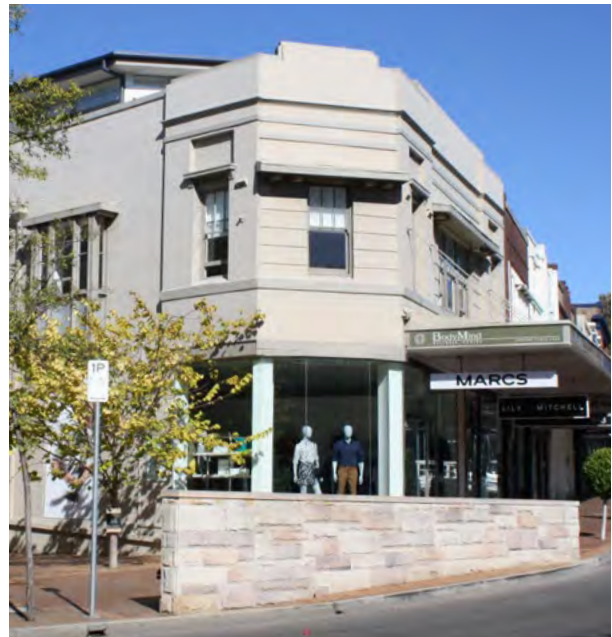
Example of an increased setback to the upper floor and a solid parapet balustrade that helps the building to 'read' as a two storey building from the street.
