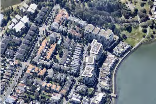
Figure K7-1 Aerial photo (source: nearmap.com)
