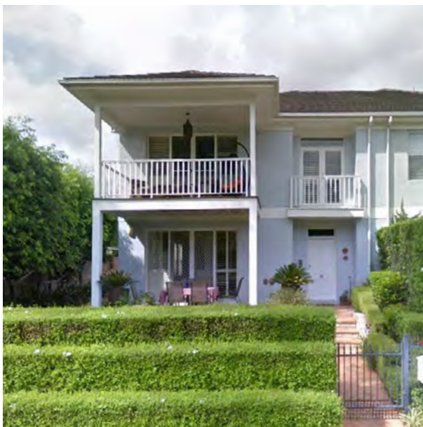
Example of a well articulated facade with the main entry, windows, balconies and a verandah clearly addressing the street
