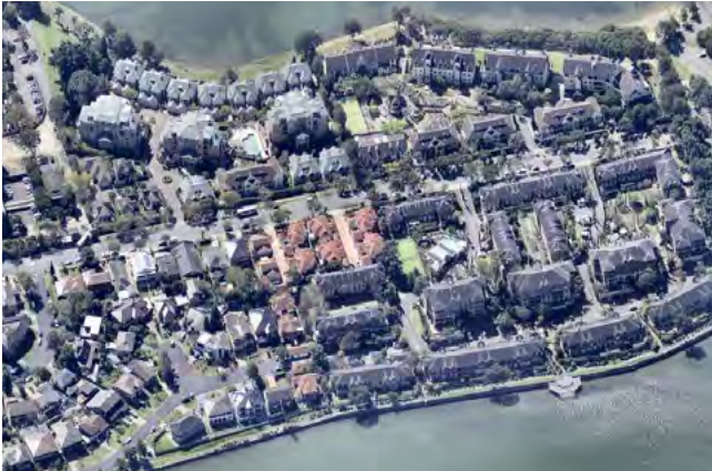
Figure K14-1 Aerial photo (source: nearmap.com)
