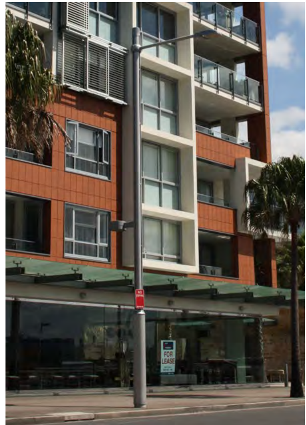
Example of balconies with a balance of solid and void in the facade composition and treatment
