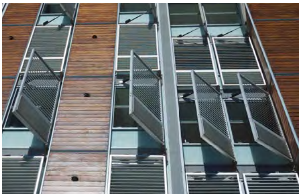
Building users should be able to open windows and operate privacy screens and sun shading devices.
