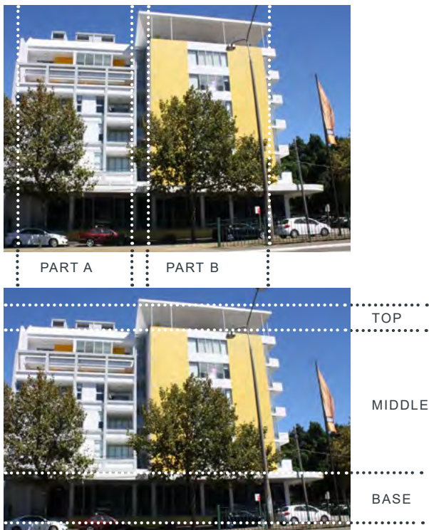
Fig G2.1 Example of a building that is vertically articulated into two components and differentiates between base, middle and top
