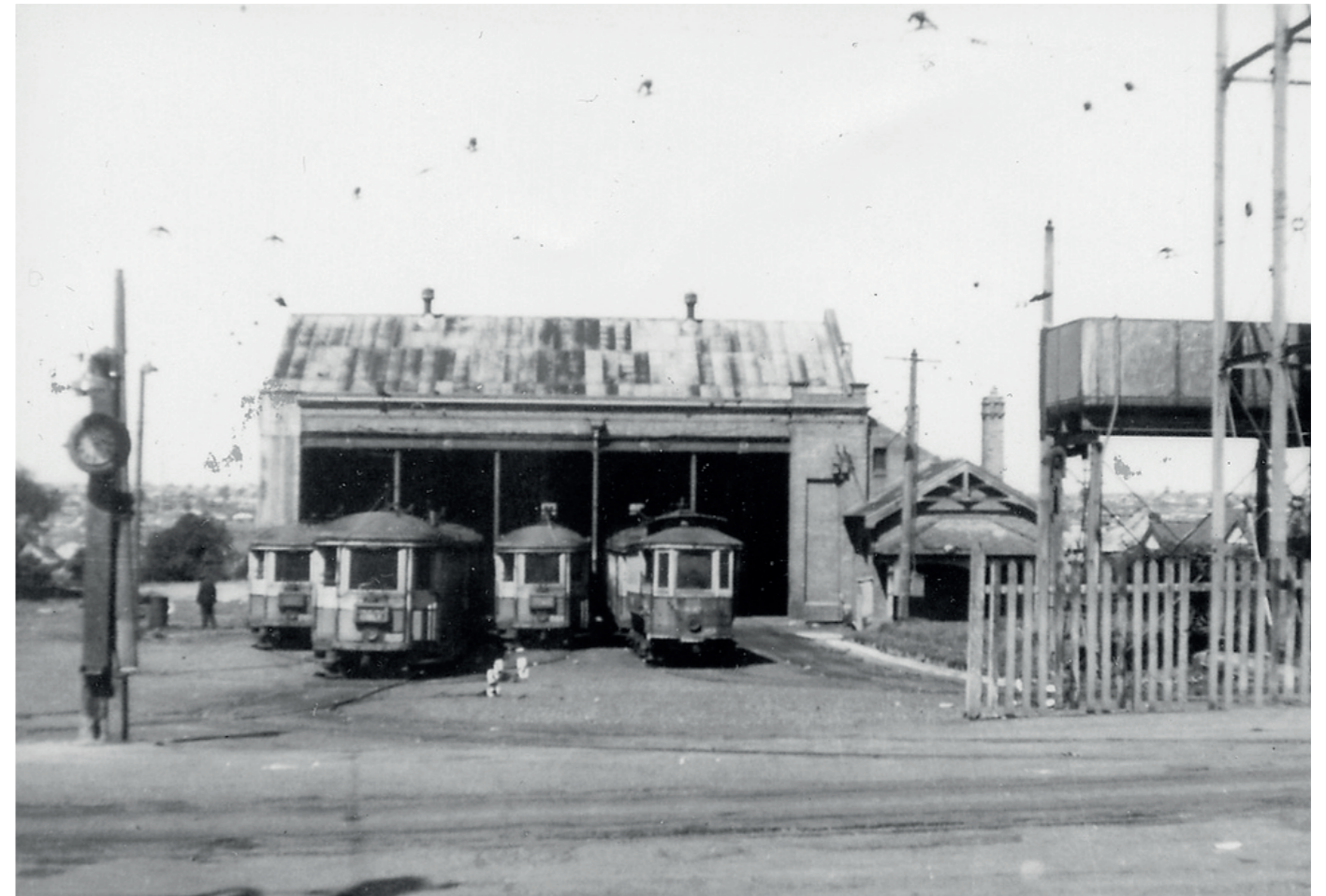
Concord Tram depot
