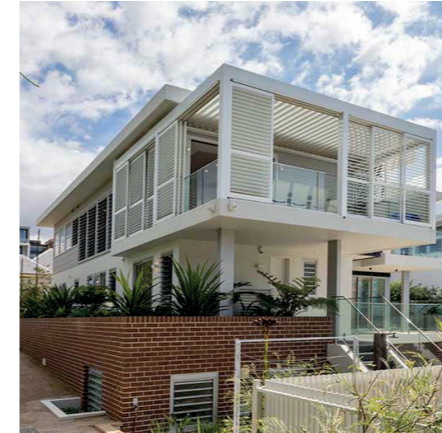
Two Storey apartment building that compliments the street character of stand alone dwellings.
