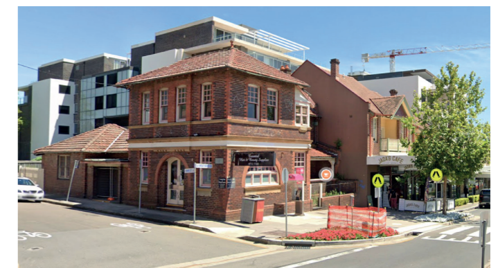
Stakeholder feedback that the new development behind Jada's Cafe on Great North Road is palatable because it retained the original building facades and the height steps back from the high street.
