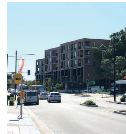
5. View looking north along Great North Road towards 5 storey RFB
