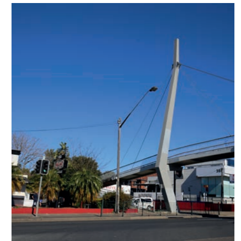
2. Pedestrian bridge over Parramatta Road
