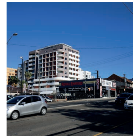
4. View looking south-west towards a 10-storey RFB
