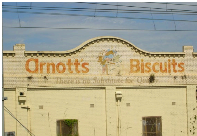
Arnott's Biscuits factory (Source: City of Canada Bay)
