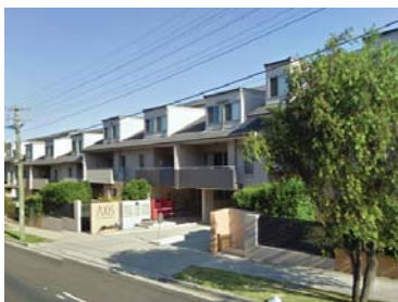
Photo 45. 57 Fairlight Street development
