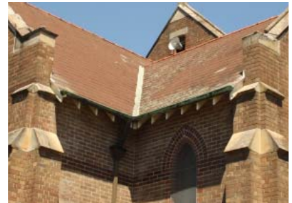
Photo 25. Detail of St. Alban's brickwork
