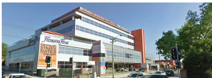
Photo 47. Commercial suites at 49 Queen Street
