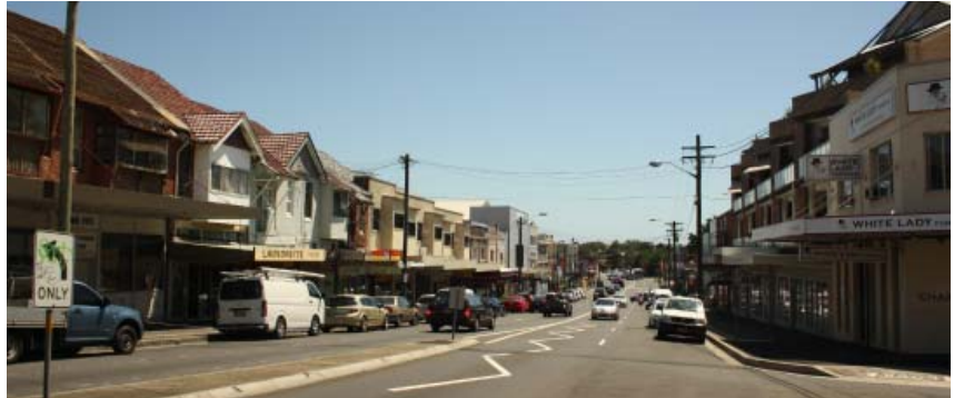
Photo 21. Both sides of the Great North Road are defined by built form, predominantly 2-3 storeys in height
