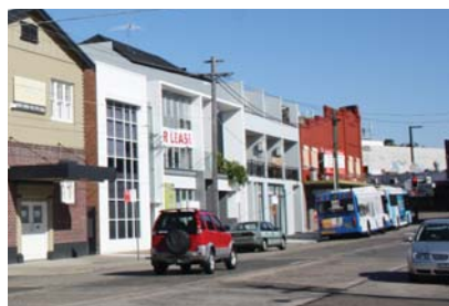
Photo 48. 181 First Avenue development
