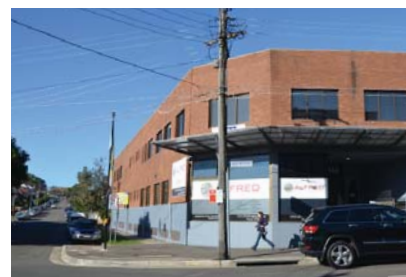
Photo 49. 144 Great North Road development
