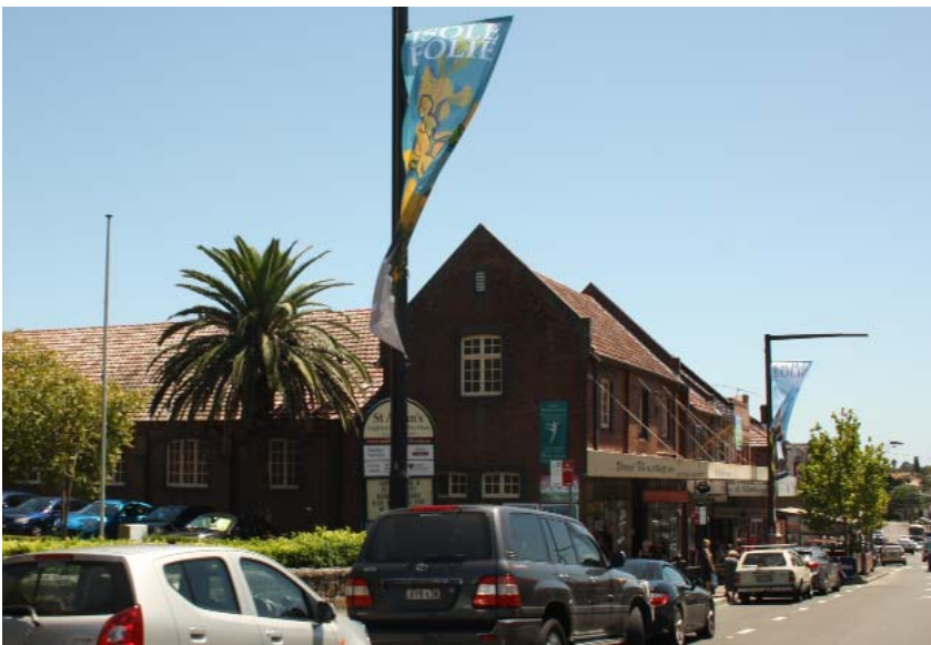
Photo 33. St Alban's Church Hall and Shops
