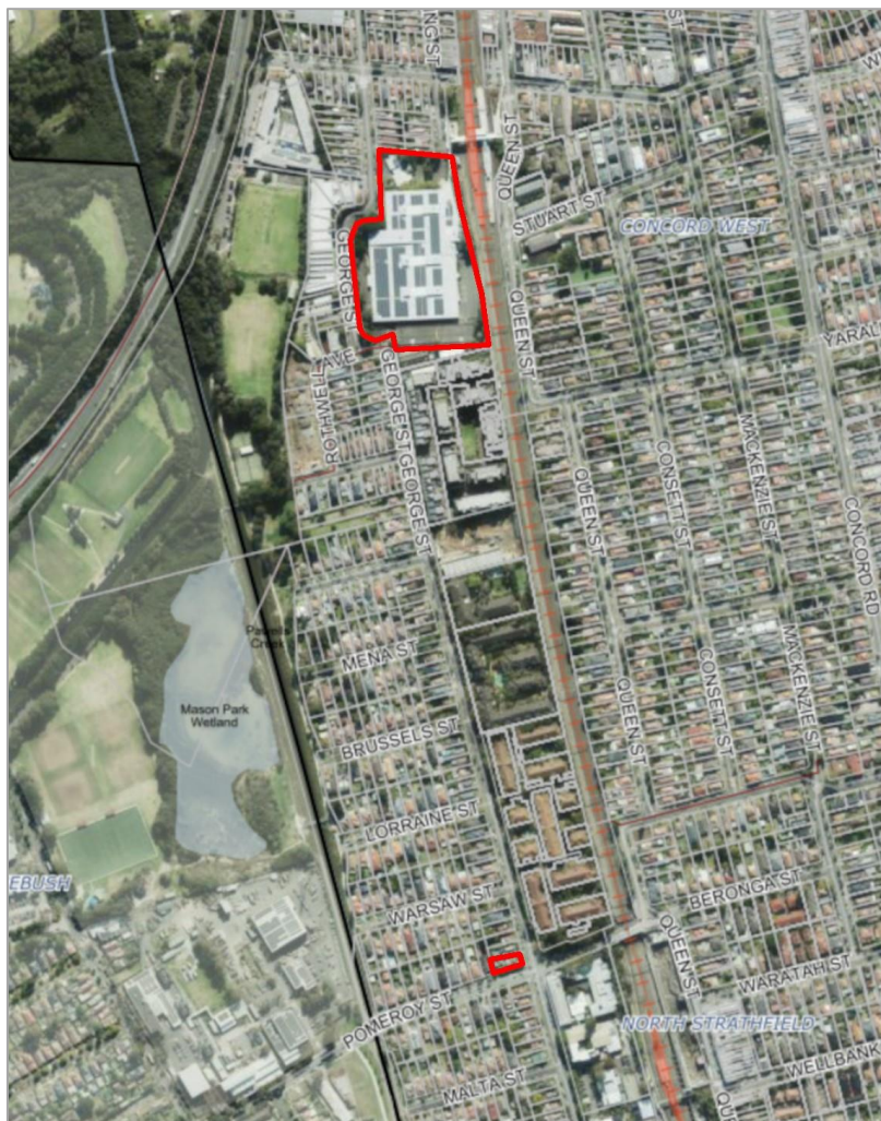
Figure 2: The Site and land at 88 George Street, North Strathfield – aerial photograph (Source: Council mapping)
