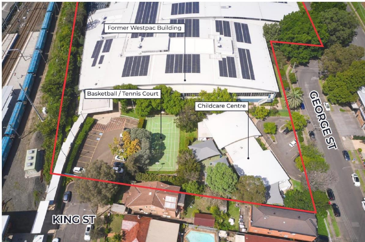
Figure 4: Existing development on site – looking south (Source: Proponent Planning Proposal)
