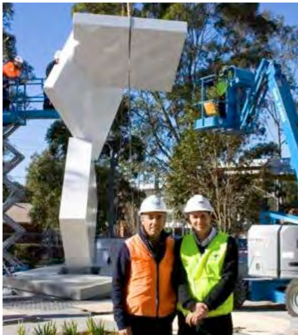
Image: Construction of 'Cumulus' by Stuart Green.
