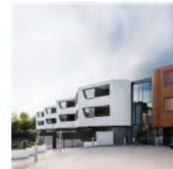
Three storey development that is appropriate in suburban area.
