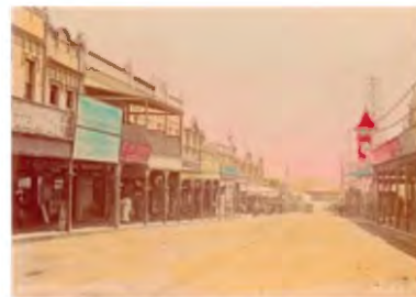
Burwood Road, Burwood
