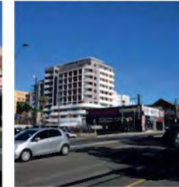
4. View looking south-west towards a 10-storey RFB
