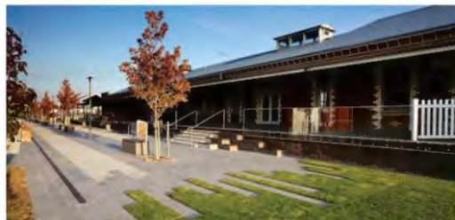
Station forecourt and plaza on Queen street to be upgraded and expanded
