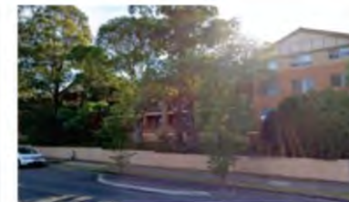
Example of an existing 3-4 storey building on George Street with a green setback to the street and deep soil planting supporting mature trees (screening the building)
