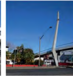
2. Pedestrian bridge over Parramatta Road
