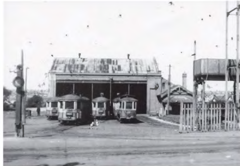
Concord Tram depot
