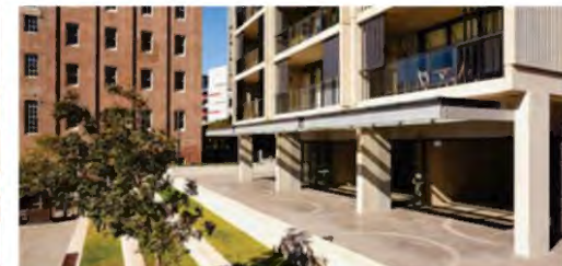
Warehouse facade preservation and sympathetic integration of new development.
