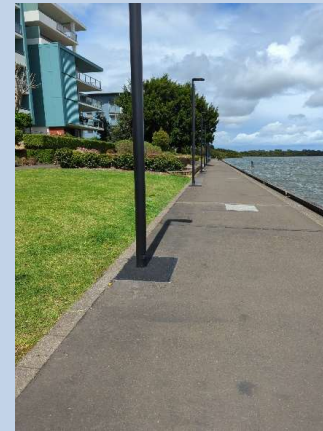
Rhodes foreshore lighting installation completed.
