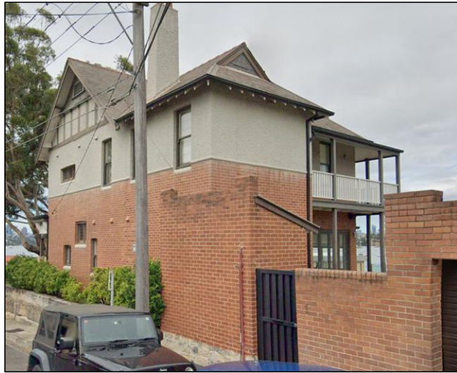
Figure 35: No. 1 Wolseley Street adjacent to the east of the subject site.
