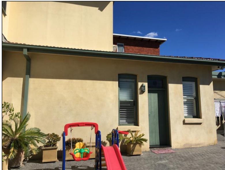
Figure 14: The main entry door.
