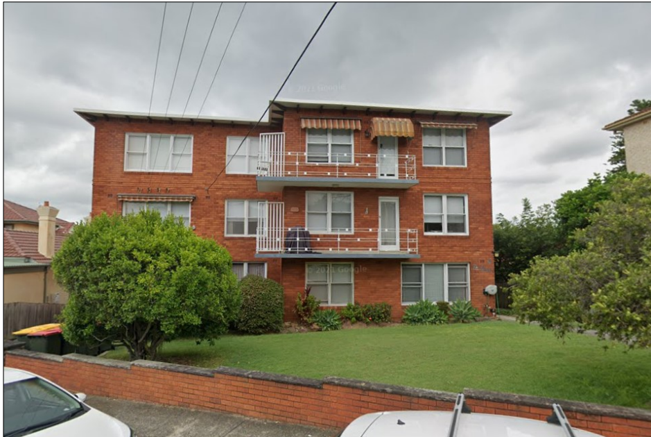
Figure 7: 5 Wolseley Street, a 3 storey residential flat building which neighbours the subject site to the south.
