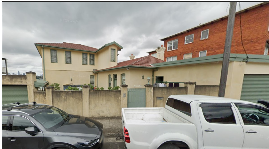
Figure 4: Front of the subject site as viewed from Wolseley Street.
