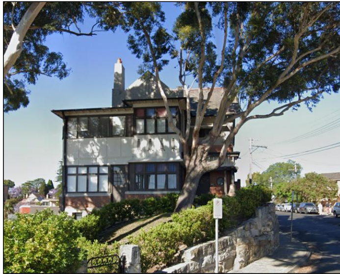
Figure 47: Looking towards the subject dwelling from the east along Walseley Street.
