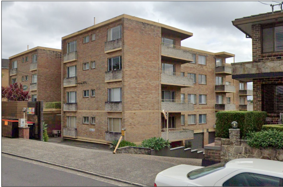
Figure 11: 6 Wolseley Street, 4 storey residential flat building located across the road.
