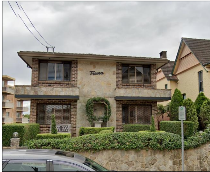
Figure 37: No. 6 Wolseley Street opposite the subject site to the north.
