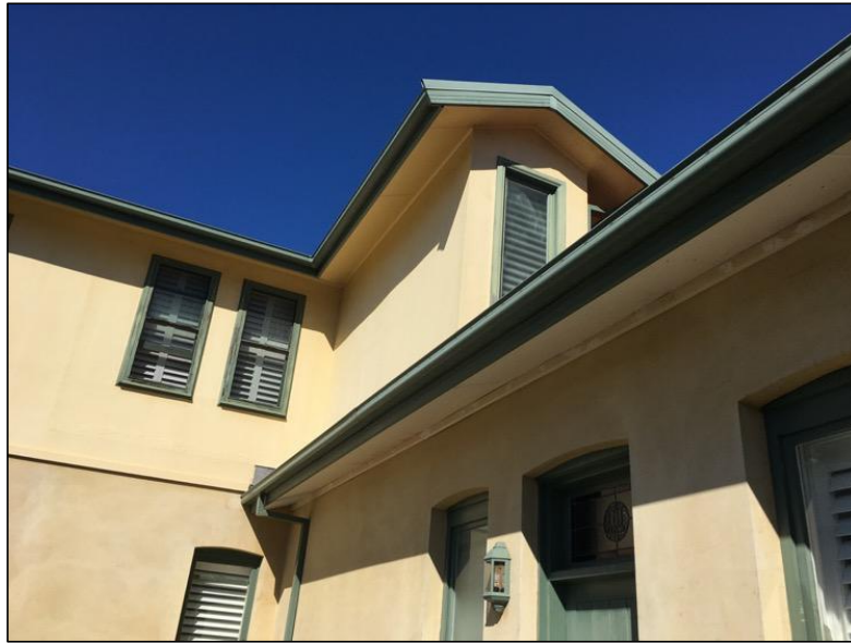
Figure 13: The gable to the first-floor.
