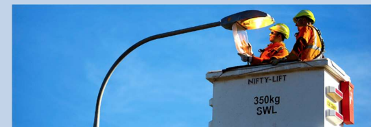
Ausgrid LED program 97% completed. Photo credit: Ausgrid.
