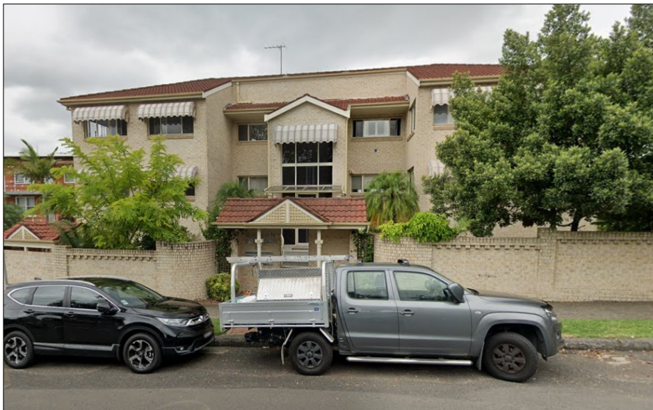
Figure 12: 5 Raglan Street, a 3 storey residential flat building located further east of the site.
