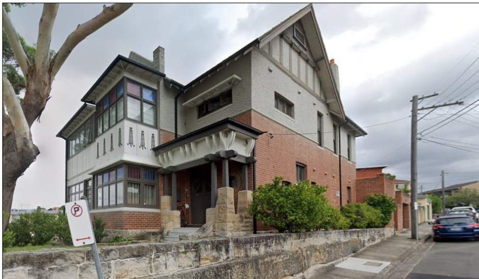
Figure 8: 1 Wolseley Street, a 2 storey dwelling house located to the east of the site.
