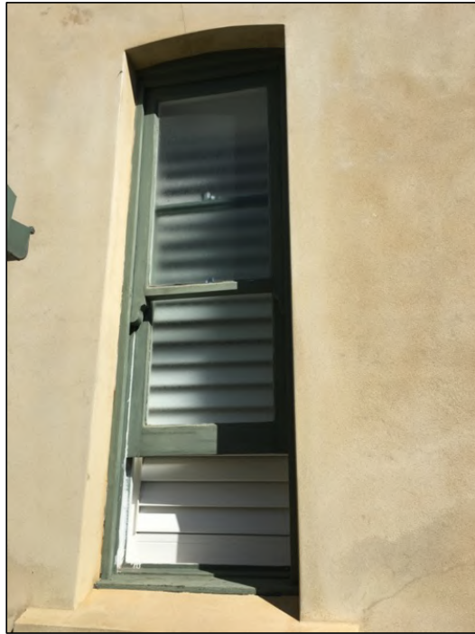
Figure 17: The only original window to the dwelling.
