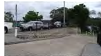
Marina driveway ramp too steep for DDA-compliance - limiting access to eastern turf terrace and foreshore
