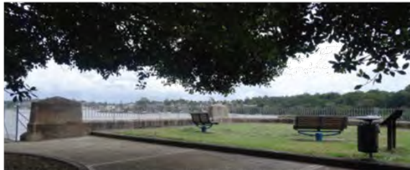
Gladesville Bridge abutment terrace space with carved capital stonework
