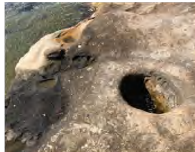
Old pier holes in existing sandstone shelves
