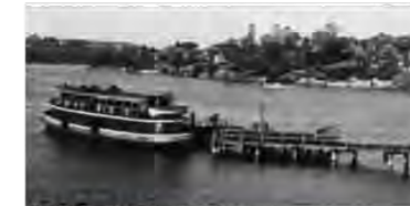
Old Gladesville Bridge ferry wharf
