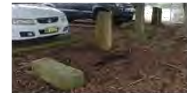
Old sandstone blocks being used as vehicular bollards, stone reflects blockwork of the remnant abutment
