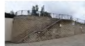
Marina stair access and driveway ramp
