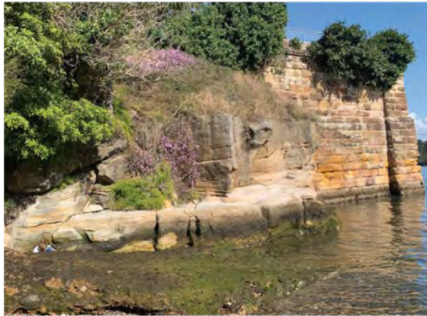
Sandstone outcrop and remnant Gladesville Bridge abutment
