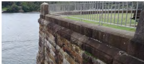
Western edge of abutment
