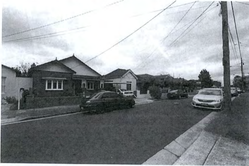
Figure 1: 9-11 Courland St, Five Dock.
