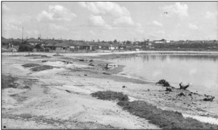
Figure 5 Reclamation works at Timbrell Park 1941
