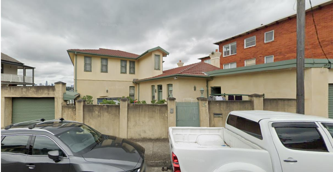
Figure 5: Current view of dwelling from Wolseley Street looking east
