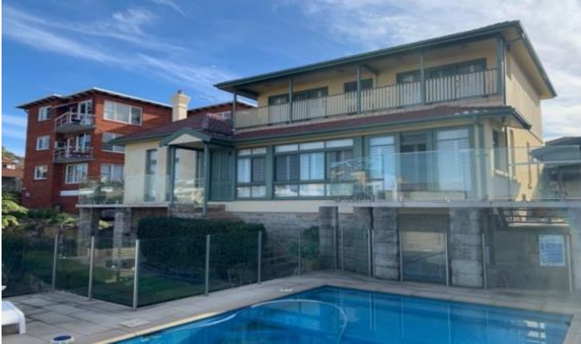
Figure 7: Rear wing of subject dwelling from St Georges Crescent
