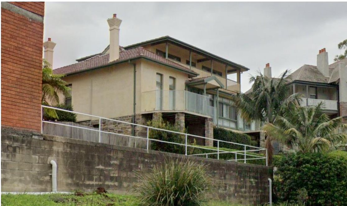
Figure 6: Current view of dwelling from St Georges Crescent looking north-west
